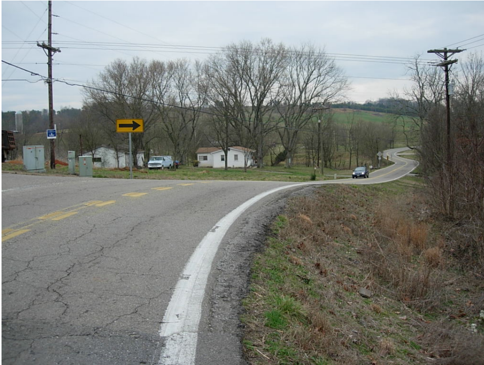
Photo 4: Reconstruct State Route 336 with a 45 mph Horizontal Curve (view looking south along SR 336)
