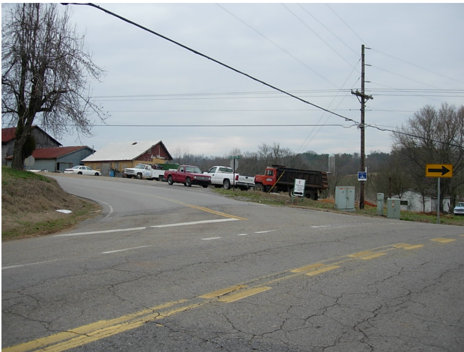
Photo 5: Existing Utilities at SR 336 and Old Niles Ferry Pike (view looking south east from SR 336 toward the intersection of Old Niles Ferry Pike)
